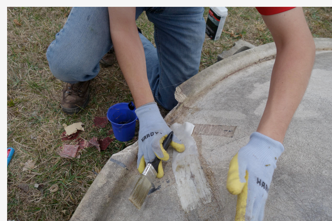
Figure 5. After cleaning and sanding the surface, cracks and the damaged edge of the dish were repaired using fiberglass cloth and automotive fiberglass resin. While at Bell Observatory, the steel support hardware was measured and inspected for bends and corrosion.
