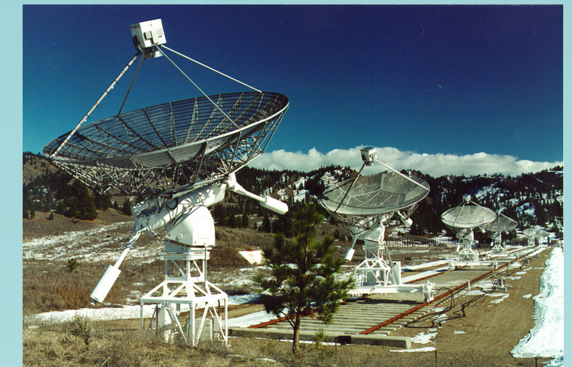
The Dominion Radio Astrophysical Observatory Synthesis Telescope, an interferometer array made up of seven connected radio dishes in British Columbia, which was used to observe the Canadian Galactic Plane Survey data used in the analysis.
