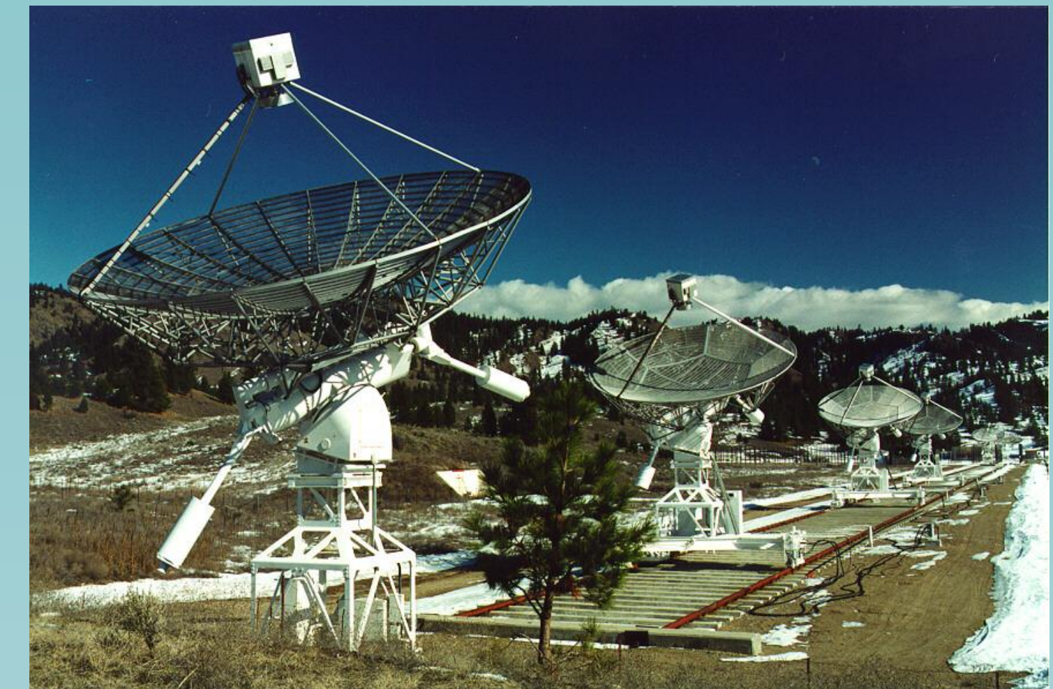
The Dominion Radio Astrophysical Observatory Synthesis Telescope, an interferometer array of 7 radio dishes in British Columbia used to observe the Canadian Galactic Plane Survey data used in our analysis.
